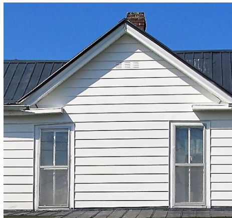
Figure 42. Storm windows should be full view design or match the window's meeting rail. See guideline 4.6.3.
