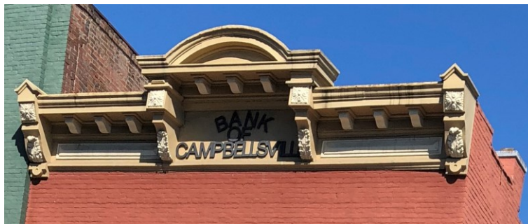
Figure 55. Original cornice elements shall not be removed or obscured. See guideline 6.5.1.
