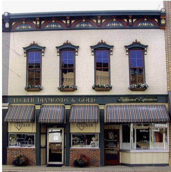
Figure 26. Raised details may be enhanced by color to highlight the features. See guideline 2.2.4.b.
