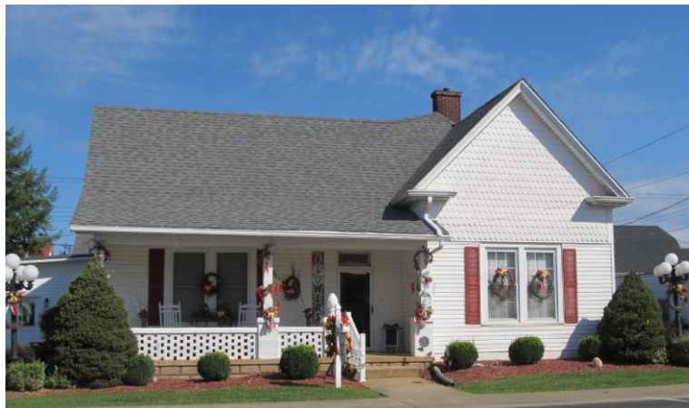
Figure 31. Clean, repair, prime and paint wood siding every five to ten years. See guideline 2.4.2.
