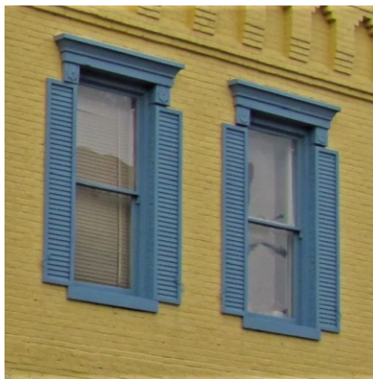
Figure 43. Shutters may be painted to contrast with the building's color and may match the color of the window trim. See guideline 4.7.2.c.
