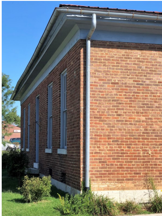
Figure 53. Replace historic gutters and downspouts with similar materials, design, dimensions and color. See guideline 6.2.1.d.
