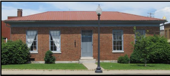
OLD TAYLOR COUNTY CLERKS' OFFICE North Columbia Avenue
