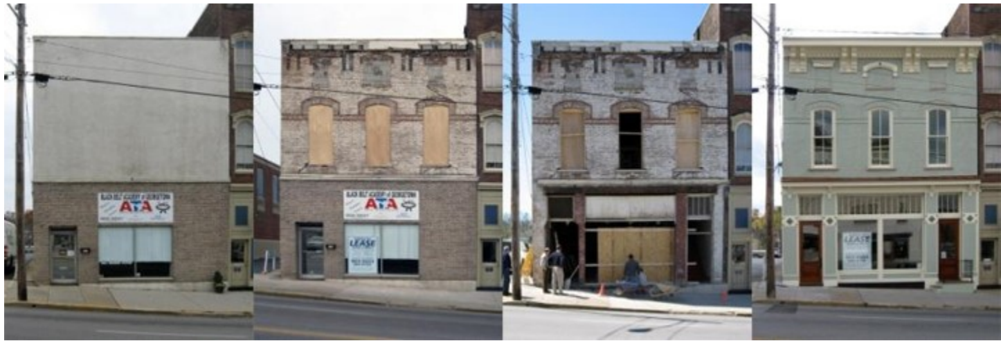
Pullen Building, Georgetown, before and after rehabilitation
