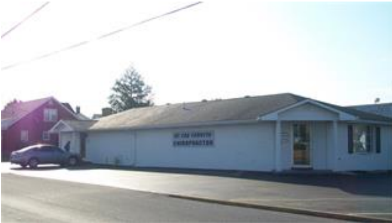
Caption: TAC396_04 The west (side) of the building with main entry on the corner of the building facing Lebanon Avenue.
