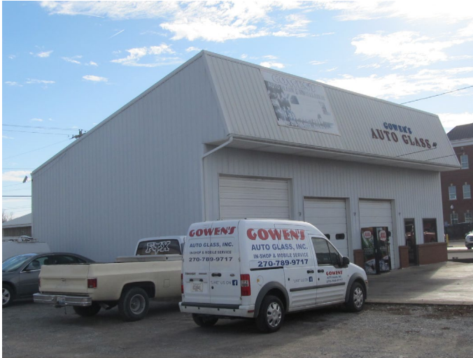
Caption: TAC408_03 A east (side) and North (front) of the building with three overhead doors, an entry door and storefront windows facing E. Main Street.
