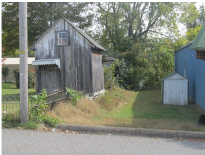
Caption: TAC436.1_01 TAC-436B North (front) and West (side) elevations of outbuilding.
