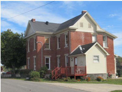
Caption: TAC436_04 TAC-436A Partial North (side) and West (rear) elevations.
